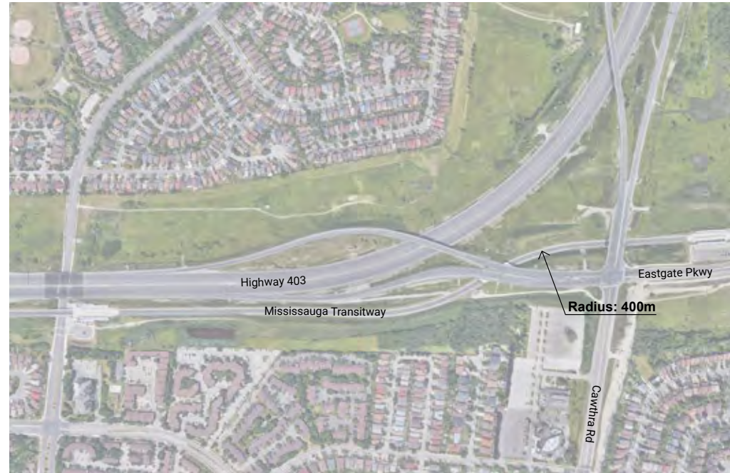
Mississauga Transitway - Highway 403 at Cawthra Road
